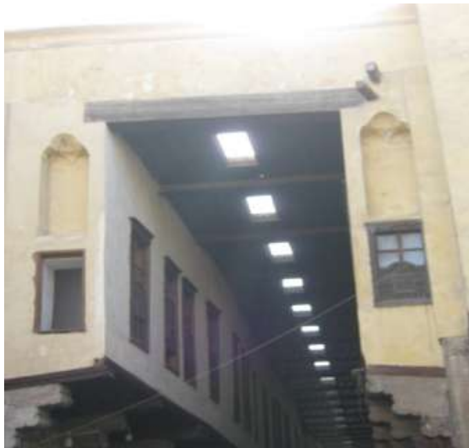
Figure (9). Wkallah Radwan Al-Fakari. After restoration processes.
