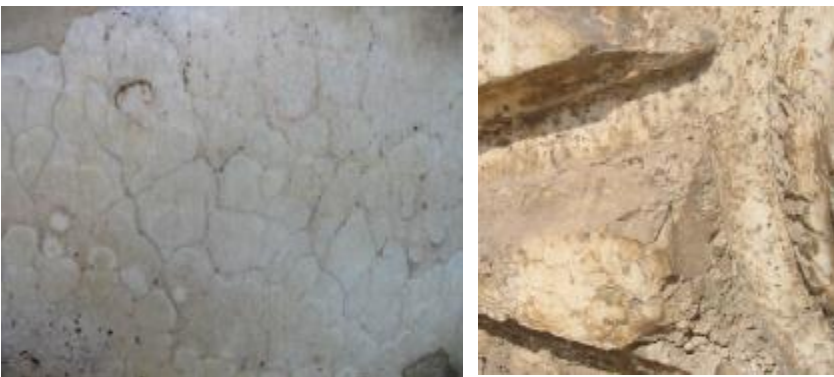
Fig.157-158 Display fissures independent of stone structure in Egyptian alabaster of both chapels at Karnak (left) and Muhammad Ali Mosque (right).
