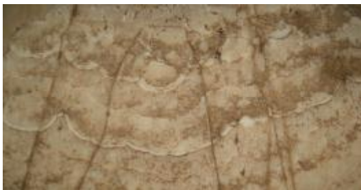
Figs. 55- 60 Display the Egyptian alabaster (Travertine) surfaces of chapels of Karnak of Wadi El-Assiuty characterized of presence of botryoidal or colloform structure and the planes of the colloform structure are weakness planes because of the tendency to break along these planes (arrows) , also display covering the convex and the outer surface of stone with a thin layer of red iron oxide and that indicts it belongs to The 3 rd type of the colloform structure forms which is of colloidal origin and existence of the spheroidal surfaces - which due to surface tension phenomena
