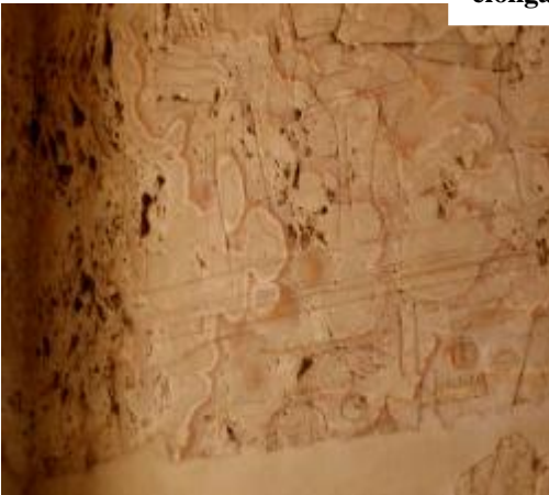
Fig. 72 display the vugs occur elongated is of the milky white type surfaces of the travertine of chapels at Karnak of Wadi El-Assiuty (it looks like weathering out of stone components clearing out of stone components
