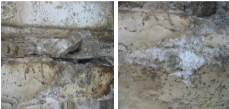
Figs.139-140 display Egyptian alabaster of the façade of Muhammad Ali Mosque displays, where display symptoms of Efflorescence Sub florescence of Halite salt
