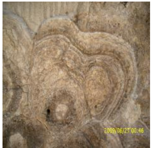
Figs.128 -131 display the travertine of chapels at Karnak of Wadi El-Assiuty, where show symptoms of Efflorescence Sub florescence of Halite salt, we can observe in the lower left photo. The form light - colored crust of salt tracing the surface where compact deposit, light - colored, changing the morphology of alabaster surface , due to mainly precipitation process .
