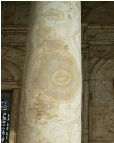
Figs.82-90 Display the difference between color of the wall-casings of Egyptian alabaster inside (interior veneers) Muhammad Ali Mosque (left column) and outside it (exterior veneers) (left column) is not only noticed but also very obvious and the Bleaching of the latter is visible , Where the coloring of honey , pale-orange , pale yellow , brown or pale tan to yellowish white with an orange tint are bleached or to white color due to exposure to the sun .
