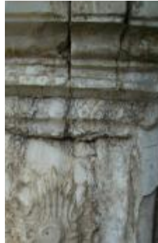
Figs. 24- 27 The short iron bars which were used to tie blocks of alabaster veneers to the wall core and were fixed in walls with lead , the rusting and corrosion of hundreds thousands of caused expansion consequently produced forces which in turn created tension resulting in the 1 st type cracks , also I have to cite that the alabaster veneer were felled by their own dead overweight .
