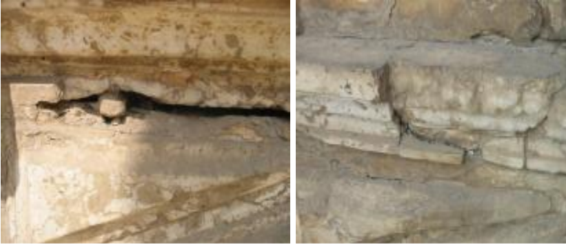
Figs. 154- 155 Display the crumbling which is Detachment of larger , compact stone elements in the form of crumbs, in Egyptian alabaster of Muhammad Ali Mosque and not observed in chapels at Karnak.
