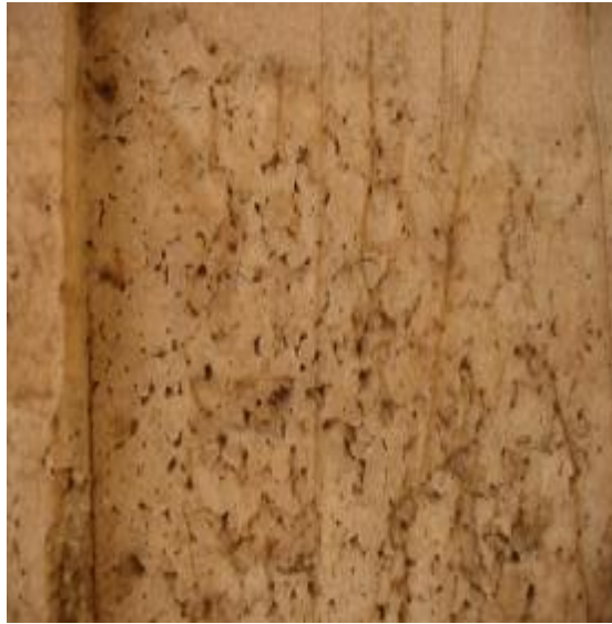
Figs. 74-75 Display superficial coarsening and granulation on the surfaces of the travertine of chapels at Karnak smoothed by corrosion polishing as external deterioration factors.
