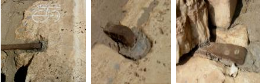
Figs. 24- 27 The short iron bars which were used to tie blocks of alabaster veneers to the wall core and were fixed in walls with lead , the rusting and corrosion of hundreds thousands of caused expansion consequently produced forces which in turn created tension resulting in the 1 st type cracks , also I have to cite that the alabaster veneer were felled by their own dead overweight .
