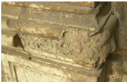
Figs. 148-149 Display Back weathering due to loss of scales where is observed in Egyptian alabaster surfaces of both chapels at Karnak (above) Muhammad
