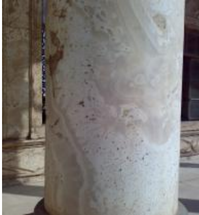
Figs.82-90 Display the difference between color of the wall-casings of Egyptian alabaster inside (interior veneers) Muhammad Ali Mosque (left column) and outside it (exterior veneers) (left column) is not only noticed but also very obvious and the Bleaching of the latter is visible , Where the coloring of honey , pale-orange , pale yellow , brown or pale tan to yellowish white with an orange tint are bleached or to white color due to exposure to the sun .
