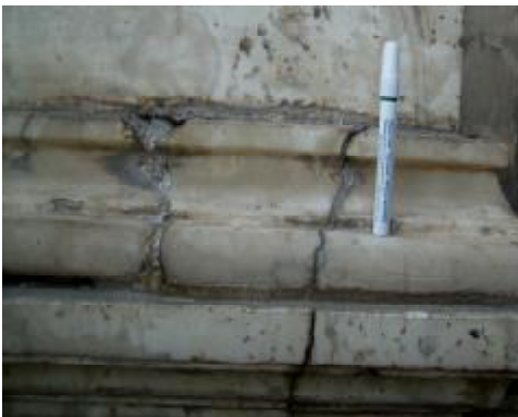
Figs. 28-31 the first type of cracks which are usually short and isolated involving small deformation of masonry , and they are distributed randomly and irregularly over the whole building - is related to both the physical and chemical properties of materials and constructional methods
