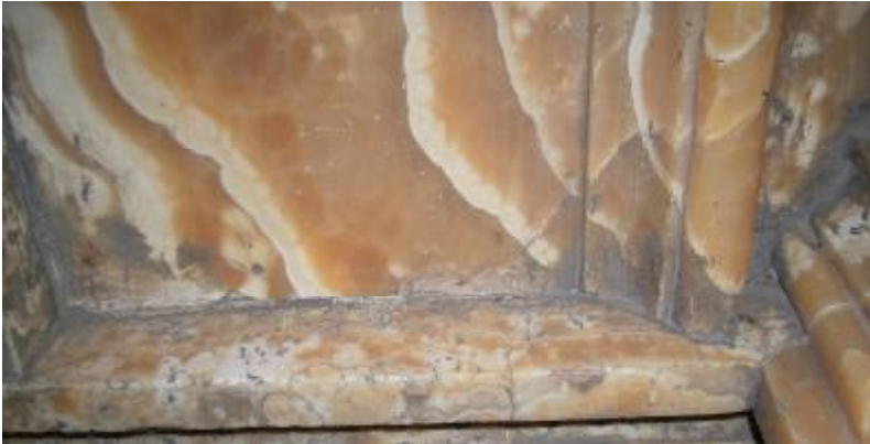
Figs. 61-64 Display the Egyptian alabaster (Travertine) surfaces of Muhammad Ali Mosque of Wadi Sannur characterized also of presence of botryoidal or colloform structure but the planes of the colloform structure are not weakness planes such as chapels of Karnak of Wadi El-Assiuty, even in external veneers , and that indicates to that weakness due to structural and geological reasons
