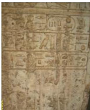
Figs.150 -153 Display the granular disintegration which is Detachment of individual grains or small grain aggregate into grus where there is detachment of larger grains as individual grains or small grain aggregates (stone grus), in Egyptian alabaster of both
