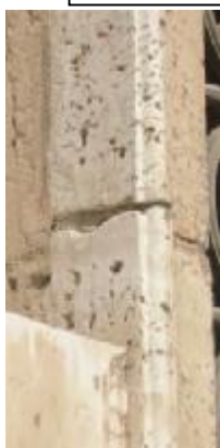
Fig. 143 lay the roughening in the travertine of chapels at Karnak as a finest relief resp. alteration of gloss due to the loss smallest stone particles or corrosion of stone surface smoothed by sawing , grinding or polishing , it is observed on the surfaces of the travertine of chapels at Karnak .
