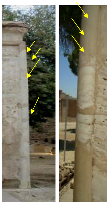
Figs. 43- 47 Display frailty and debility structure of some ornamental architectural elements of Egyptian alabaster chapels at Karnak such as the Cavetto Cornices and torie which are along the horizontal upper edge and along the corners of the façade of them , in addition to being hanged partially on space , have exposed them to fracture and loss or to erosion (arrows) .
