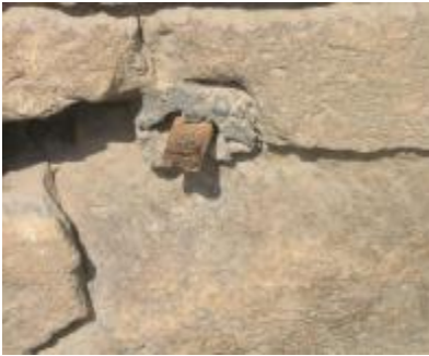
Figs. 24- 27 The short iron bars which were used to tie blocks of alabaster veneers to the wall core and were fixed in walls with lead , the rusting and corrosion of hundreds thousands of caused expansion consequently produced forces which in turn created tension resulting in the 1 st type cracks , also I have to cite that the alabaster veneer were felled by their own dead overweight .
