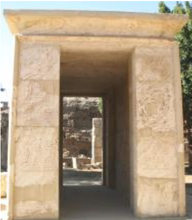
Figs. 91- 95 Display the Bleaching of the exterior surfaces of the chapel of Thutmosis IV at Karnak and other adjacent alabasterite chapels Where the coloring of honey , pale-orange , pale yellow , brown or pale tan to yellowish white with an orange tint are bleached or faded to white color due to exposure to the sun .
