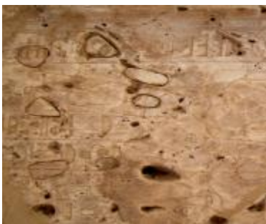
Fig.73 display the vugs repair in the surfaces of the travertine of chapels at Karnak of Wadi El-Assiuty
