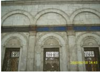
Figs.82-90 Display the difference between color of the wall-casings of Egyptian alabaster inside (interior veneers) Muhammad Ali Mosque (left column) and outside it (exterior veneers) (left column) is not only noticed but also very obvious and the Bleaching of the latter is visible , Where the coloring of honey , pale-orange , pale yellow , brown or pale tan to yellowish white with an orange tint are bleached or to white color due to exposure to the sun .
