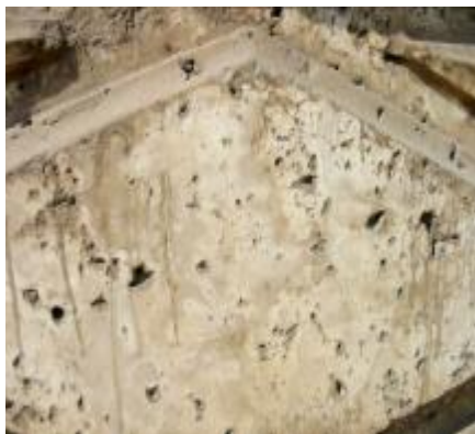
Figs.144-147 Display the form of small pits - are caused by biogenically induced corrosion processes, particularly in carbonate rocks , it is noticed only on the Egyptian alabaster surfaces of Muhammad Ali Mosque , it is not noticed on the surfaces of chapels at Karnak
