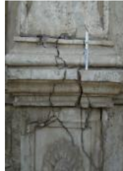
Figs. 28-31 the first type of cracks which are usually short and isolated involving small deformation of masonry , and they are distributed randomly and irregularly over the whole building - is related to both the physical and chemical properties of materials and constructional methods
