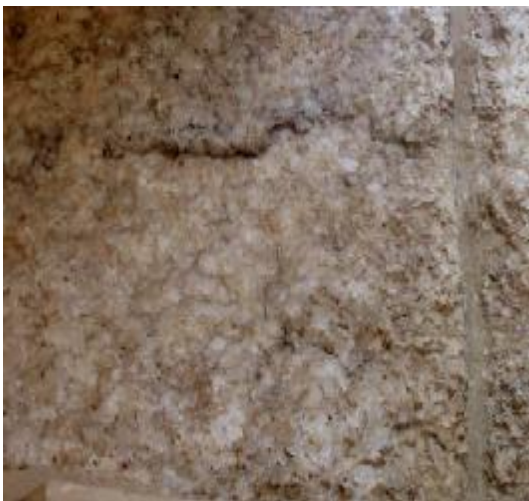
Fig. 143 lay the roughening in the travertine of chapels at Karnak as a finest relief resp. alteration of gloss due to the loss smallest stone particles or corrosion of stone surface smoothed by sawing , grinding or polishing , it is observed on the surfaces of the travertine of chapels at Karnak .
