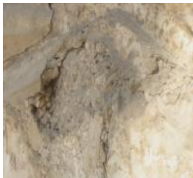
Figs. 148-149 Display Back weathering due to loss of scales where is observed in Egyptian alabaster surfaces of both chapels at Karnak (above) Muhammad
