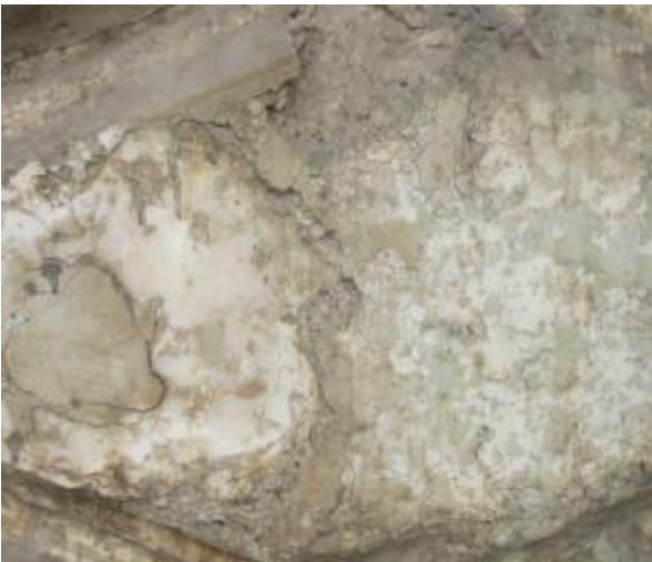
Figs. 154- 155 Display the crumbling which is Detachment of larger , compact stone elements in the form of crumbs, in Egyptian alabaster of Muhammad Ali Mosque and not observed in chapels at Karnak.
