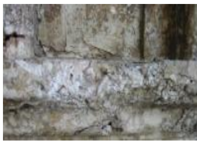
Figs.150 -153 Display the granular disintegration which is Detachment of individual grains or small grain aggregate into grus where there is detachment of larger grains as individual grains or small grain aggregates (stone grus), in Egyptian alabaster of both
