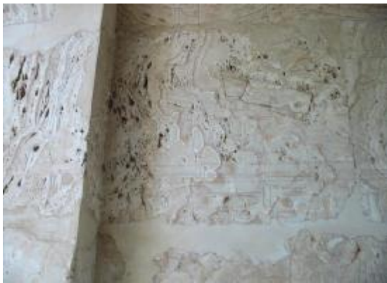
Figs. 91- 95 Display the Bleaching of the exterior surfaces of the chapel of Thutmosis IV at Karnak and other adjacent alabasterite chapels Where the coloring of honey , pale-orange , pale yellow , brown or pale tan to yellowish white with an orange tint are bleached or faded to white color due to exposure to the sun .
