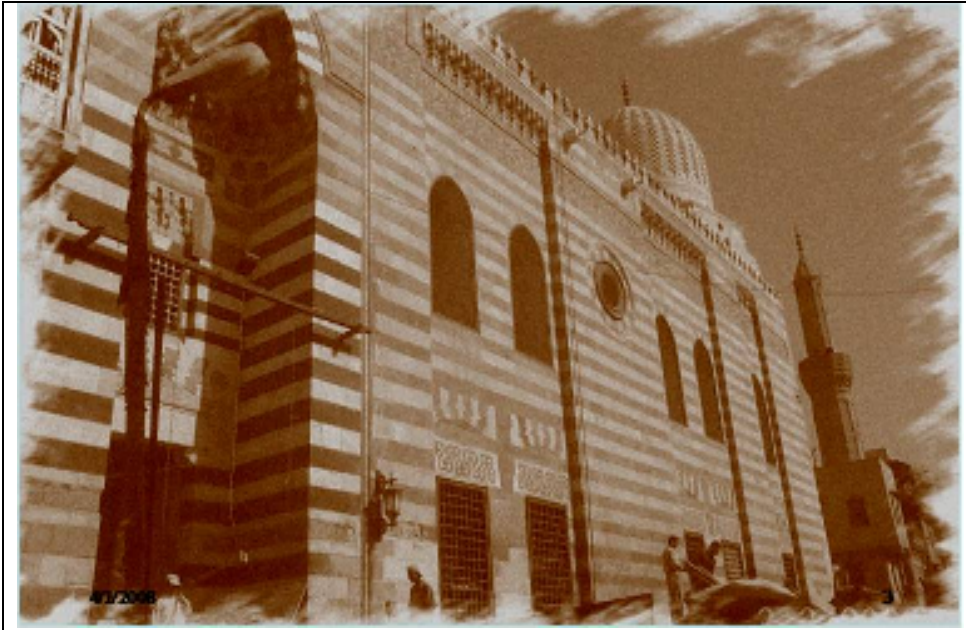
Fig.1 shows the main façade of Al- Ashraf Bersbay Madrasa .
