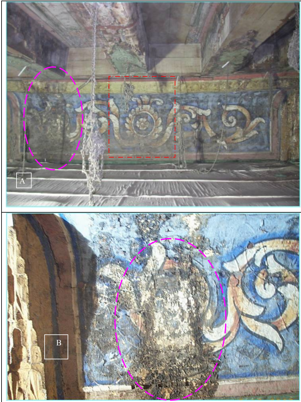
Fig.8 A, B., Shows, details from the Q.C. decoration of Al Ashraf Bersbay Madrasa and its very bad status.
