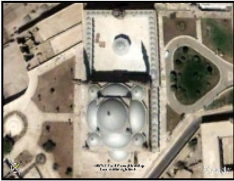
Plate (2): Aerial-View of Moh. 'Ali Mosque; shows the compound domed roof (After: Google Earth Website).
