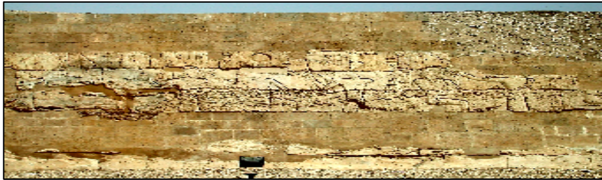
Fig.63) displays the weak and partial lost north wall of the Seti I temple at Abydos which are subjected to mechanical pressure and moistured & polluted soil , rubbish and garbage of the outraged urban context ,so it was compensated with an alternate stone of low permeability and high hardness from Eisawy limestone..
