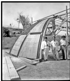
a) Trying the cutting out of lead plates for covering dome surfaces.
