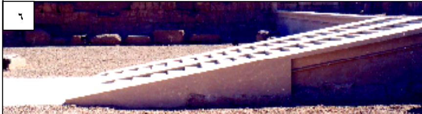
Fig.63) displays the weak and partial lost north wall of the Seti I temple at Abydos which are subjected to mechanical pressure and moistured & polluted soil , rubbish and garbage of the outraged urban context ,so it was compensated with an alternate stone of low permeability and high hardness from Eisawy limestone..
