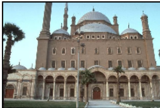
Plate (5): N-W Façade of Moh. 'Ali Mosque; shows the external arcade topped by shallow domes and covered with alabaster clad.
