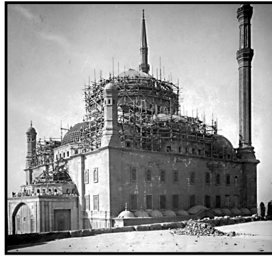
e) Reinforcement and frameworks of domes before casting concrete.
