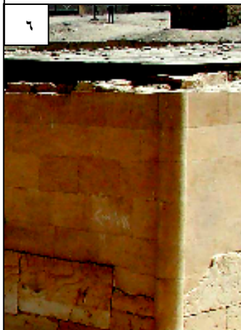
Figs.64 - 65) display the compensation with plastic repair (mortars) for the cavetto cornices , torie of the terrace of the second court and edges of staircases and balustrades of the staircases leading from the first to the second court of the temple of Seti I (64) and Ramesses II (65) at where the plastic repair is more suitable for formation and reconstruction of many of the ornamental and architectural elements with accuracy and homogeneity plus the possibility of addition of chemical additives to mortars to increase resistance of friction of the infantry, also prevents from disturbing fragile areas .
