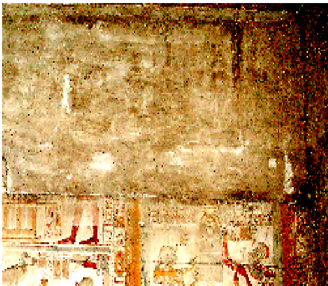
Figs .10-11 Display examples of emergency for partial reconstruction with the original stone from the local quarry for preventive conservation where the seven chapels of the temple of Seti I at Abydos had lost their ceilings and big parts of their upper walls , so the partial reconstruction restored esthetical role and provided a preventive conservation from weathering particularly inscriptions and pigments .
