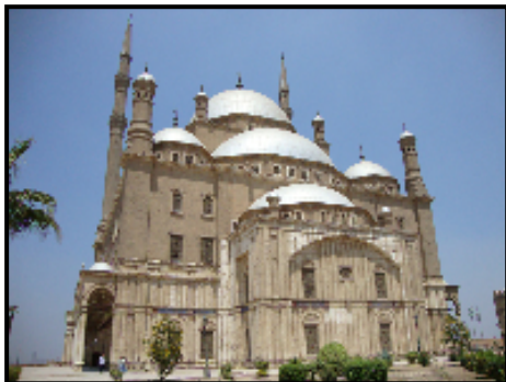
Plate (4): S-E Façade of Moh. 'Ali Mosque; shows alabaster cladding and the semi-dome over the mihrab.
