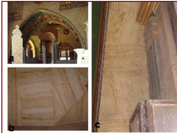
Fig. 2 shows the interiors of the main central chambers decorated with imitated marble occupied the upper parts of walls and ceilings
