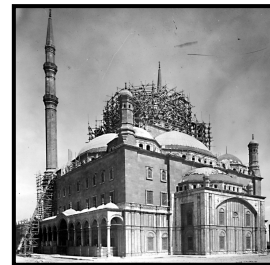
c) After casting the domes and semi-domes and before casting the central dome.
