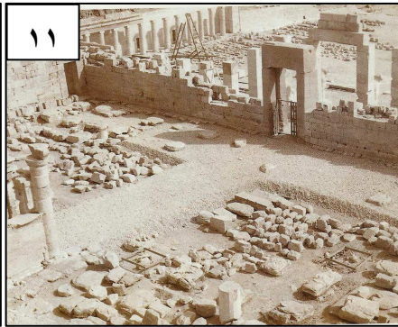
Figs. 10-11 the remains of the Upper Terrace and courtyard before the beginning of 1961 works where the thousands of blocks had been laid in rows then transported to the stores then the decoration and the texts had been traced , photographed and documented in await of reconstruction
